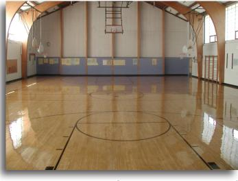
single-part formulation provides comparable durability to two-part, crosslinked finishes without the risk of catalyzing too much material that would have to be discarded. Hydrothane HT's low odor formulation is a pleasure to work with, levels well, builds quickly and dries in approximately two hours. Hydrothane HT is non-flammable, utilizes green chemistry and has a low VOC content of 150 grams/liter that complies with all current State and Federal Volatile Organic Compound Regulations.
